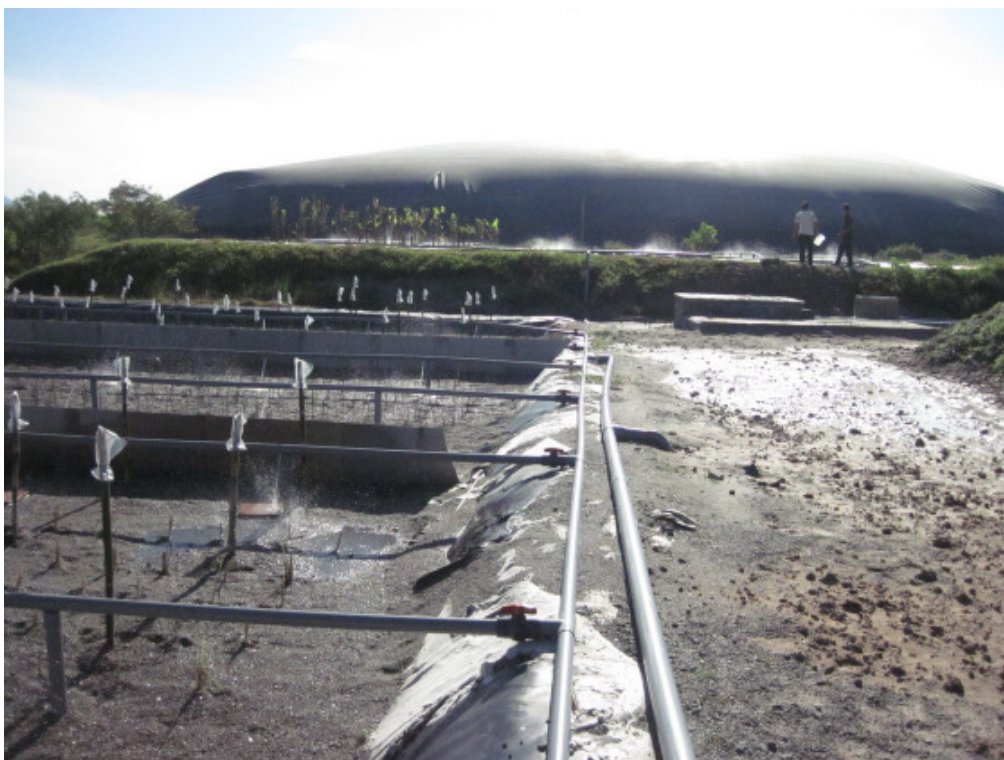
Baustelle Vietnam November 2010
